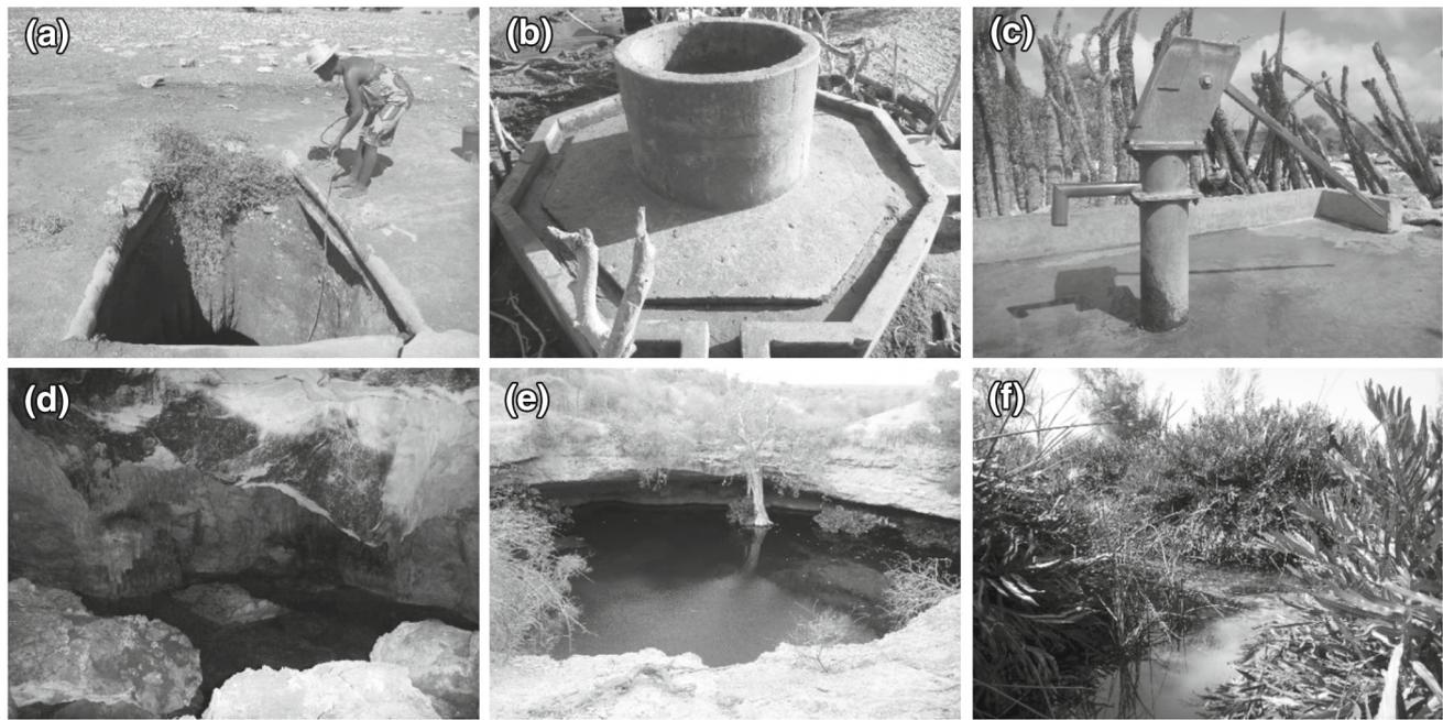
**Fig. 2** Examples of the types of water sources sampled. **a, b** Wells dug directly in the ground or reinforced with a concrete or rocks and with an uncovered outlet. Well water is drawn to the surface using a bucket
